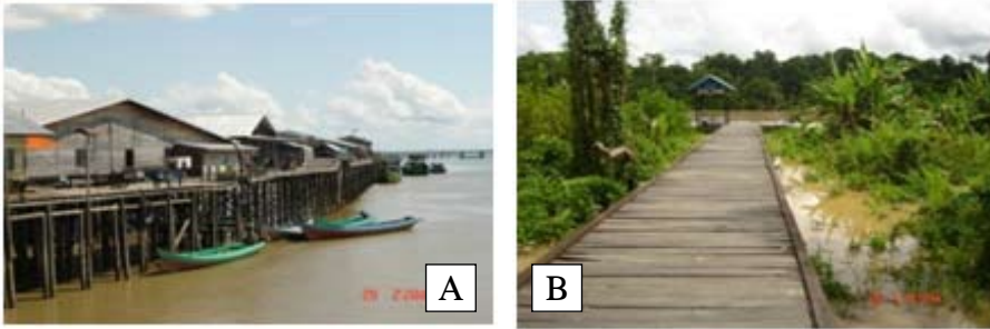
Figure 6.4. Figure 6.4 (A) House in coastal area of Balikpapan above water with ironwood pillars and posts; (B) Footpath or bridge made from ironwood timber
