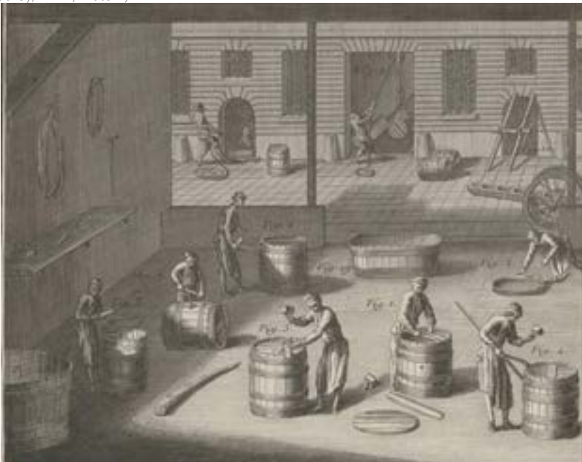
Figure 4.6: Finishing casks in an 18th-century French cooperage. Fig. 1: Measuring the headboards; Figs. 2-4: Placement of the hoops; Fig. 5: Driving hoops; Figs. 6-7: Drilling holes (Fougeroux de Bondaroy, 1777; Plate VI).
