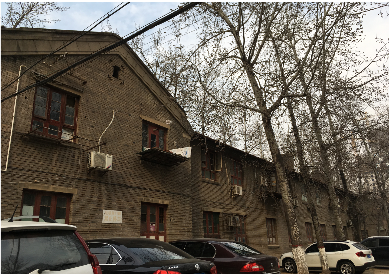
Figure 6.2: The original Soviet-style buildings. Photo taken by the author.
