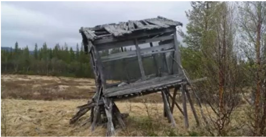
Figure 3 Structure for storage
