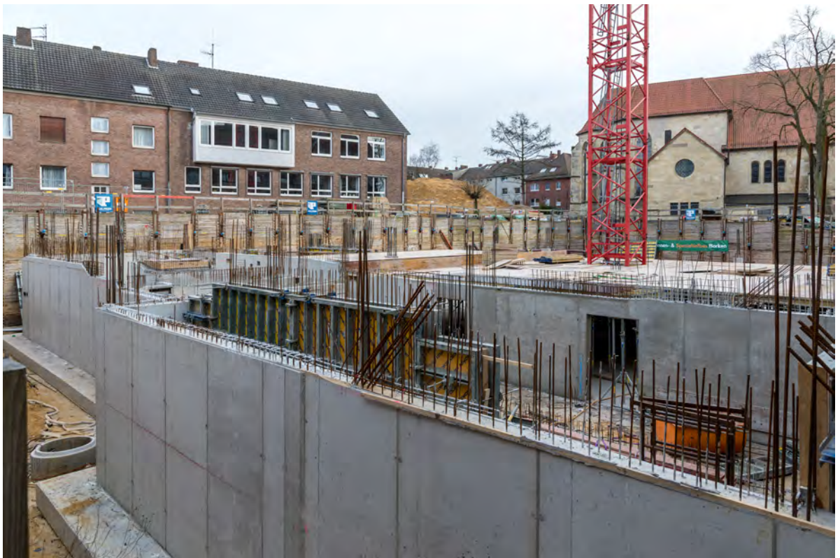
Figure 1: The image illustrates the impact of modern construction on the archaeological record, demonstrating the "tabula rasa" effect. In close proximity to the historical buildings are the subterranean foundations of the new structure, which would destroy any archaeological remains. Consequently, an archaeological excavation was initiated prior to the commencement of construction. (Intergeneratives Zentrum (IGZ) Dülmen (Germany). Source: https://www.lwl.org/pressemitteilungen/nr_mitteilung.php?urlID=33520 . (site visited on 13-12-2024). (Photo: Dietmar Rabich, https://commons.wikimedia.org/wiki/File:Dülmen,_Baustelle_IGZ_-_2018_-_1441.jpg ; https://creativecommons.org/licenses/by-sa/4.0/legalcode ).
