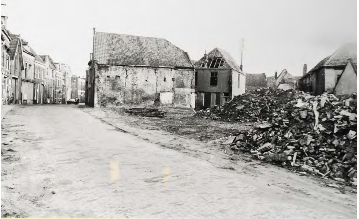
Figure 3: The Noordenberg Quarter in Deventer represents a medieval district of the city. In the aftermath of the Second World War, a considerable number of the dwellings in this locality were in a state of disrepair. The initial proposal was to demolish the entire district as part of a wider urban renewal initiative. Ultimately, following protests, only a partial demolition was carried out, which nevertheless resulted in significant disruption to the historical urban fabric. The photograph depicts the demolition of a wall of houses on Molenstraat, revealing the rear of Korte Noordenbergstraat 21. ( https://proxy.archieven.nl/0/10D8ED4A90C9766DE0504C91A40655FB ).
