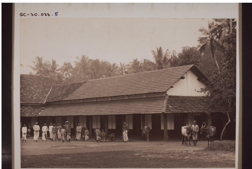
Figure 10.12: Basel Mission school in Mangalore using the Basel Mission tiles for its roofing. Source: Basel Mission Archives, Basel. 32
