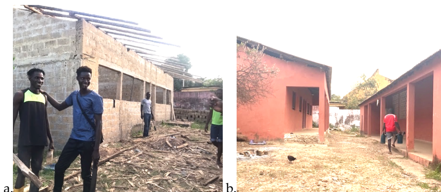
Figure 20. The second block being built from scratch by deaf men (a) in 2022, and the two buildings when ready (b) in 2024
