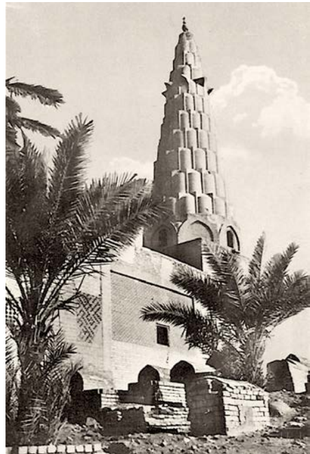
Figure 6 Zumurrud Khatun complex, exterior view
