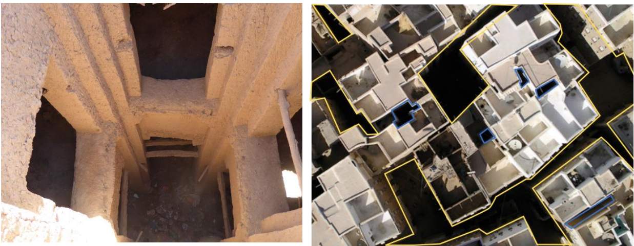
Figure 168. Air and light wells in recent architecture. Left: small central courtyard or light well in an abandoned town house, southeast Morocco (photo by author). Right: City of Shibam, Yemen. Lines indicate where light and air wells are placed. Yellow are public spaces (small squares, alleys), blue are internal light/air wells or small courtyards (photo: Shibam Urban Development project, http://archnet.org/sites/5215 . Lines drawn by author).
