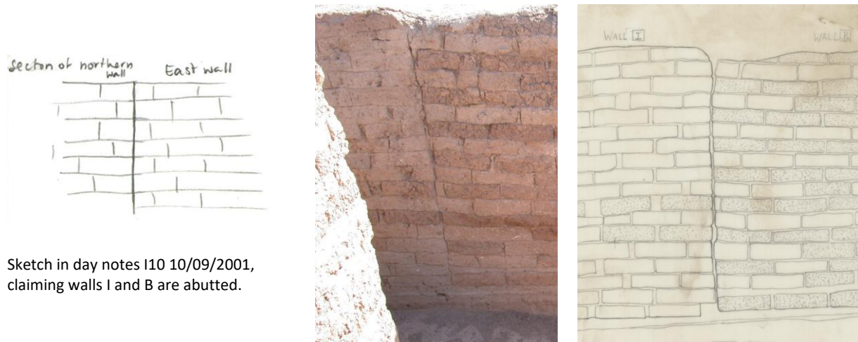
Figure 78. Abutted or bonded? All documentation of the connection of these walls suggests they were abutted. The top was disturbed by a grave, and the other side was not investigated with the same rigour. The mirroring set of walls across the central room however suggest that bonding was done by just one brick on one side of the wall (Figure 79).
