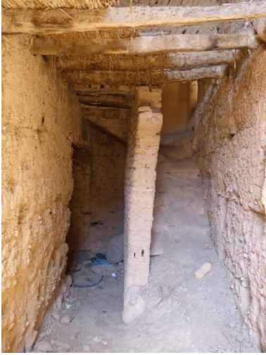
Figure 108. An example of a stair with mud brick spine wall in a ruinous house in Morocco. Like in Figure 49, the mud brick steps are put on a palm trunk base. The mud bricks have now degenerated to a precarious loam slide which the author climbed up to roof (photos by author).
