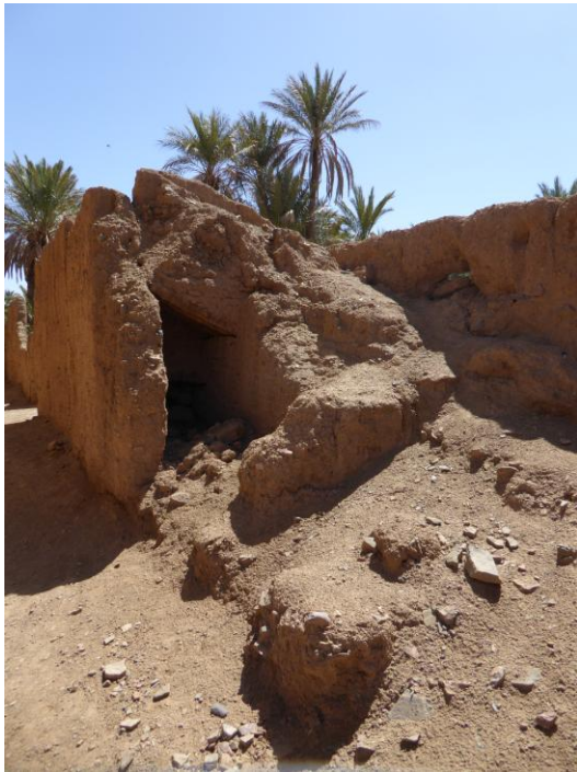
Figure 107. Ruined staircase in Morocco. The mud bricks of the steps have weathered to an unrecognizable degree. The wooden base construction still holds and protects the empty space under the stairs, but when it gives way the stairway would only be recognizable by the walls of the stairwell (photo by author).
