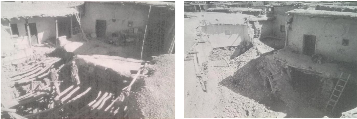
Figure 20. Demolition of a village house in the early 1980s, west Iran. Left: salvaging of roof beams. Right: the same house three years later. Much rubble is lying on the ground, but its distribution is very uneven. The house on the right is still inhabited (After Friedl & Loeffler 1994, figs.6 & 8).
