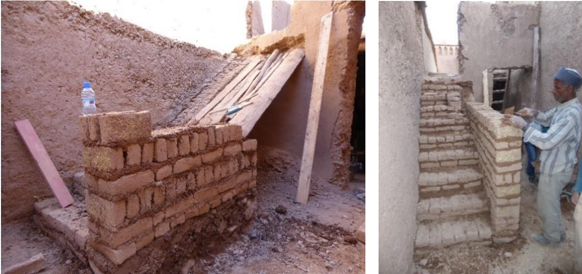
Figure 110. A stair with a solid base and retaining wall of masonry and a timber superstructure under construction in Morocco. It was constructed in just over one day by a master builder and (unexperienced) assistant (photos by author).
