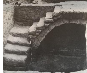
Small stairs in a house in Nippur. The single half arch is a remarkably slender construction (after McCown, 1967, Plate 48B).
