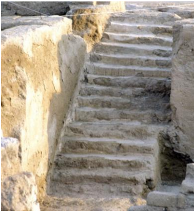
Figure 108. An example of a stair with mud brick spine wall in a ruinous house in Morocco. Like in Figure 49, the mud brick steps are put on a palm trunk base. The mud bricks have now degenerated to a precarious loam slide which the author climbed up to roof (photos by author).
