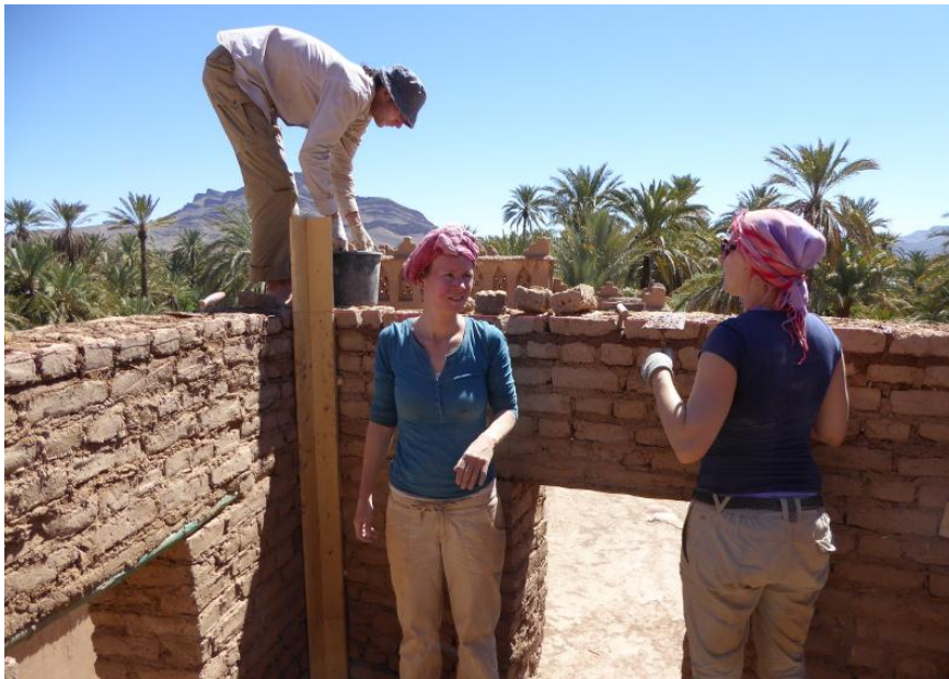
Figure 49. Bricking up a wall while standing on top of it. No scaffolding needed. Scaffolding was however regularly used on this project. This approach developed by coincidence while looking for an efficient way to finish the last part of the wall without having to adjust the scaffolding. Photo made by author during a loam construction workshop near Agdz, Morocco.
