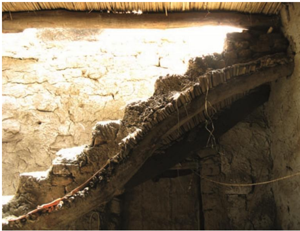
Figure 111. A variation on stair construction from Egypt. Here, just two beams form the support of the stairs, while a strong layer of reed stem mats support the mud brick steps (after Correias-Amador, 2011, p. 16).
