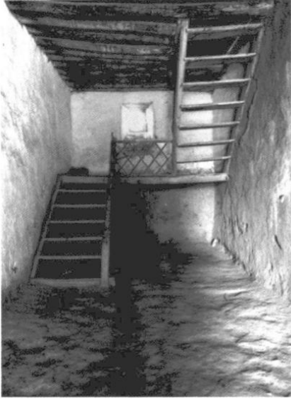
Figure 106. Timber stairs. Left: stairs in a house in Cafer Hüyük, Turkey. These U-shaped stairs are supported by a landing made of large beams embedded in the wall (after Aurenche et al. , 1997, fig. 4.13). Right: a common type of wooden stair construction. It uses so called newels, or vertical posts, to suspend the entire structure (drawing by Bill Bradley).
