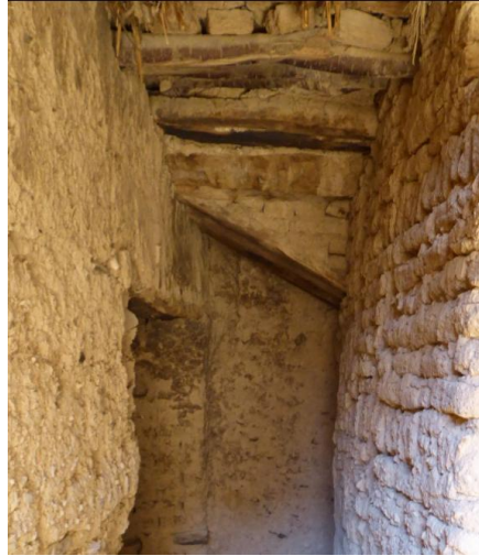
Figure 108. An example of a stair with mud brick spine wall in a ruinous house in Morocco. Like in Figure 49, the mud brick steps are put on a palm trunk base. The mud bricks have now degenerated to a precarious loam slide which the author climbed up to roof (photos by author).
