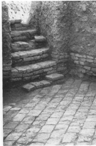
Baked brick stairs in old Babylonian Ur, unplastered. Each step is three bricks high
