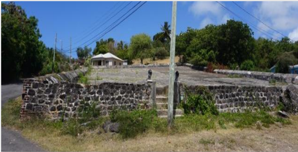
Figure 25. Historic Tank Bay Water Catchment (Antigua)
