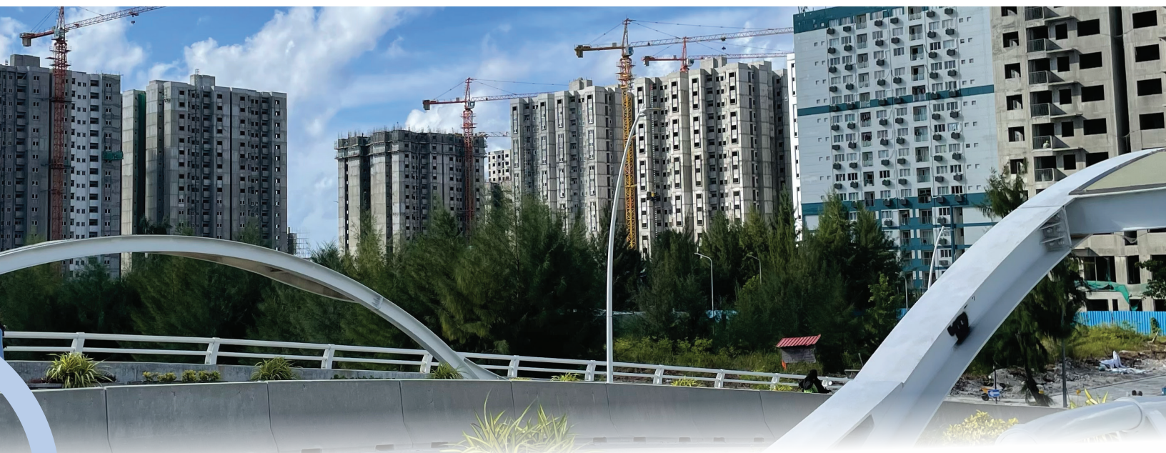
Photo: Massive construction of high-rise apartments on Hulhumalé, a reclaimed island north of Malé, the capital island city in the Maldives. Nearly all construction materials and labour come from India and China.
