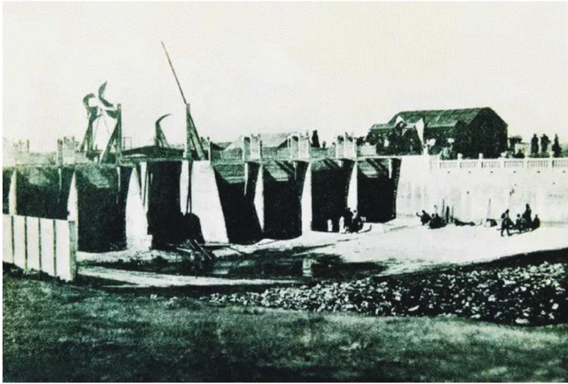
Figure 5. Yaowang Harbor Sluice during Construction. [Nantongshi gangzhaqu danganguan 南通市港闸区档案馆, and Zhangjian yanjiu zhongxin 张謇研究中心, eds., Telaike yu nantong baotan shiliao 特来克与南通保坍史料 (Historical Materials about Hendrik De Rijke and the Prevention of the Yangtze River Embankment Collapse in Nantong). Nantong, 2009].
