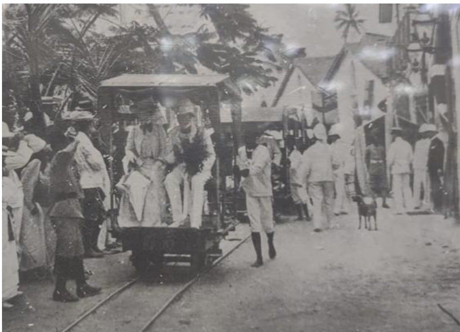
Fig 2.4 An African labourer pushing the trolley carrying Sir Charles Eliot, the governor of the Kenya colony, and Mrs Chamberlain, through the streets of Mombasa, 1904. Photo courtesy of the Kenya Railway Museum, Nairobi.
