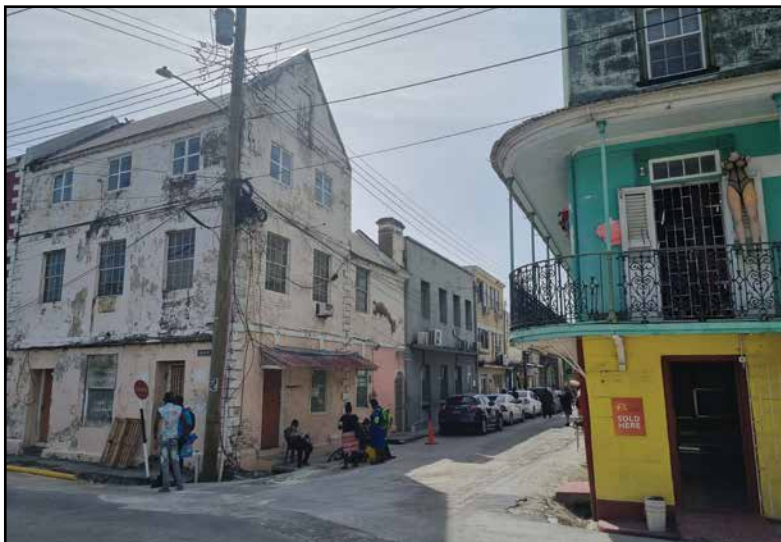
Fig. 2 One of the oldest brick buildings in Bridgetown (17th century), with a poorly thought out roof repair that has made the historic Dutch gable disappear from view (picture by De Waal, February 8, 2024).
