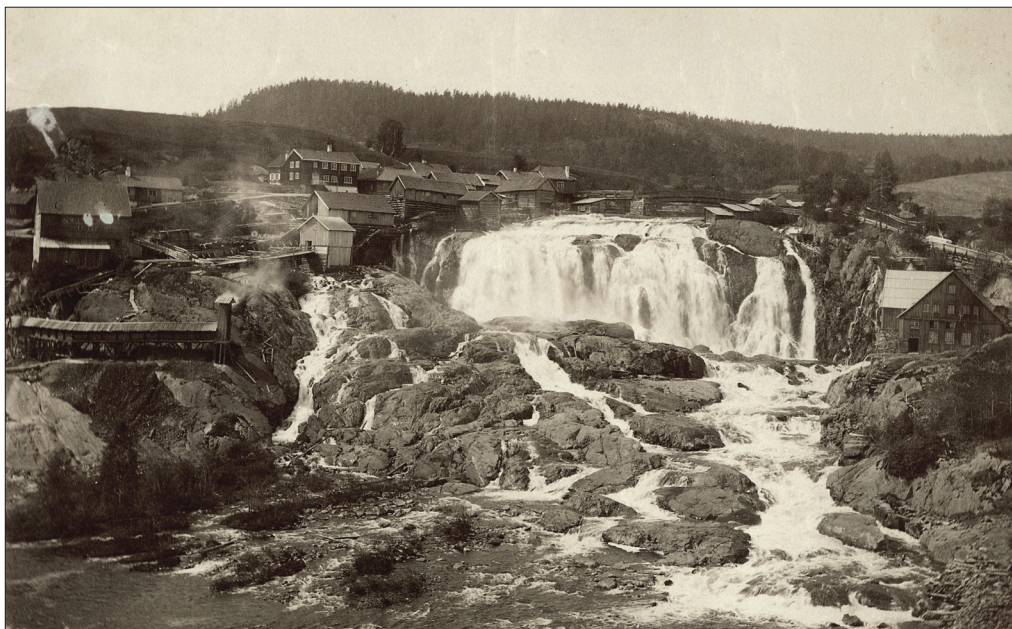
Figure 1. The Blue Colour Works in 1892, showing the waterfall Haugfoss. The building to the far left is one of the calcination huts and it is connected to the giftfang arsenic catcher (long, sinuous building ending in a short smoking chimney, just left of centre). The large building just below and right of Haugfoss is the stamping mill, powered by water from the waterfall. Copyright of Buskerud Fylkesfotoarkiv.
