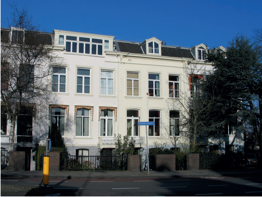
Fig. 6: Noordeindsplein. Left is no. 4a, right (bearing its construction year, 1872) no. 6a.
