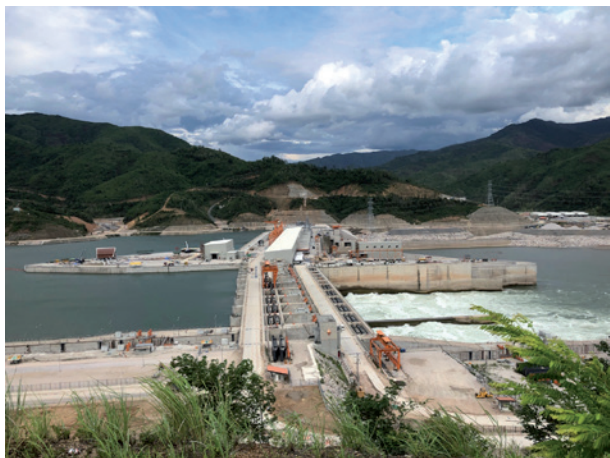
Picture 8b: Xayabury dam under construction (photo credit: Diana Suhardiman, 2019)
