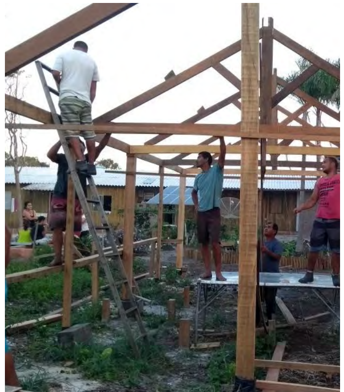
Community members build a house in Nova Enseada, their chosen relocation site. © Carolina Kotchetkoff, 2017
