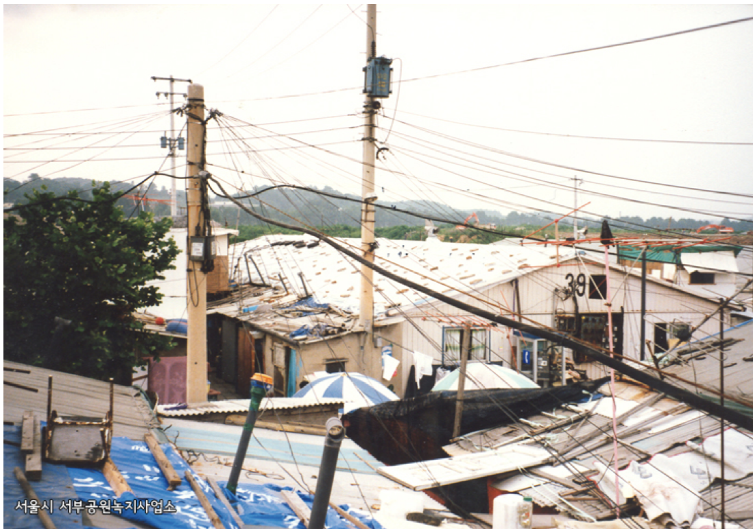
Figure 4-11 Nanjido prefabricated housing complex, tenement 39
