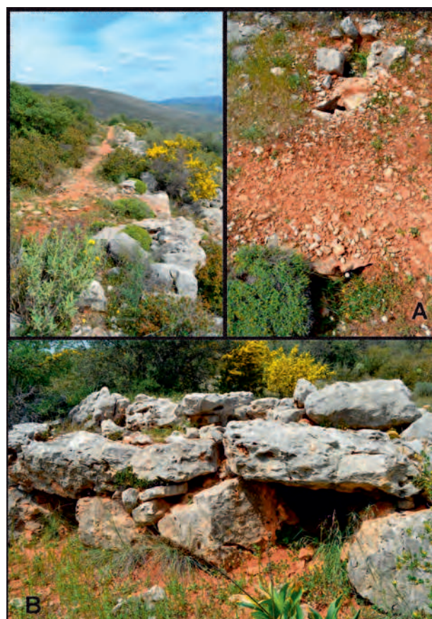
Figure 6. Section of Mycenaean road (highway 1, top left) with water management features of drainage channels (A) and multiple culverts (B) (photos Ann Brysbaert).
