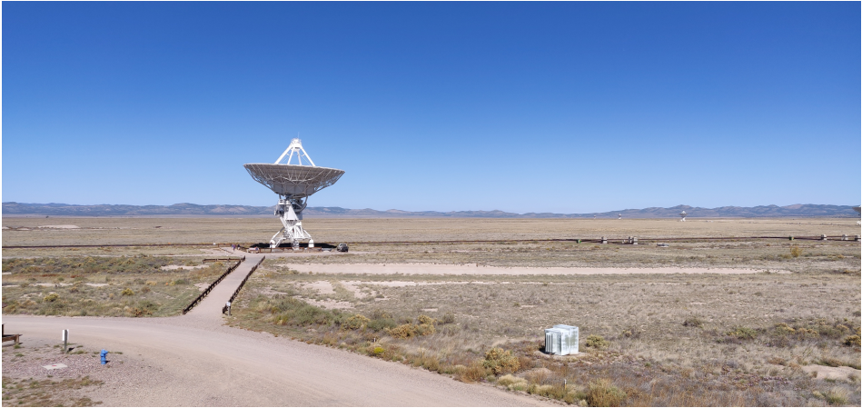
Figure 1.5: The Very Large Array in New Mexico, USA, shown in A-configuration. In the foreground, the antenna on position W08 is visible, with the Northern arm located in the background.
