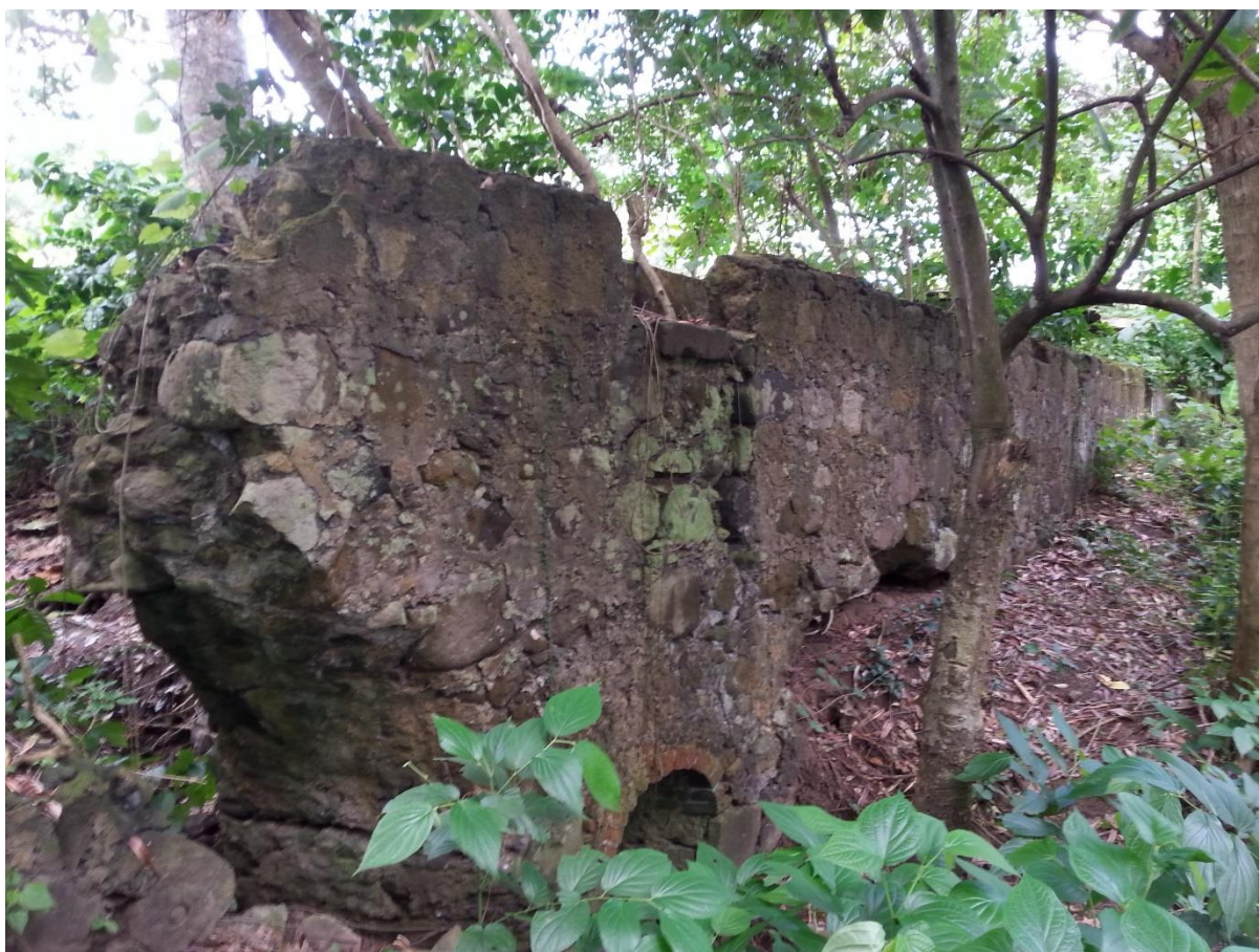
Figure 8.4 Possible ruins of the canal for the Duquesne estate along the banks of the Duquesne River, Duquesne, St. Patrick built with enslaved labor, c18 th century
