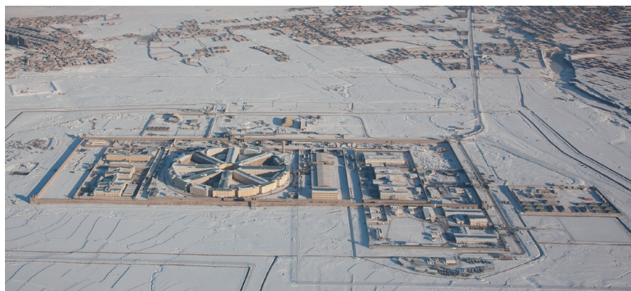
Illustration 2: Aerial view of Pul-e-charkhi prison and the surrounding area
