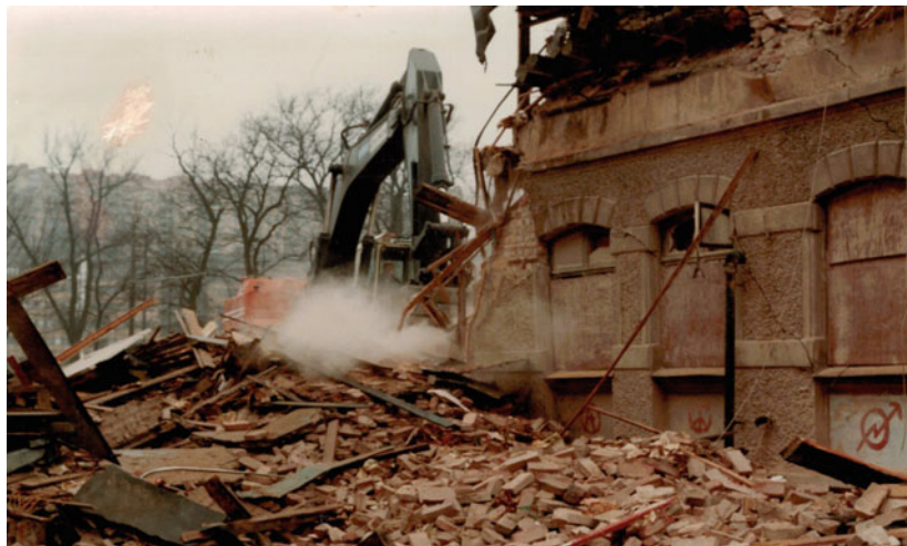
Picture 3.2 Demolition in Haga in the 1980s (Photo Salka Sandén)
