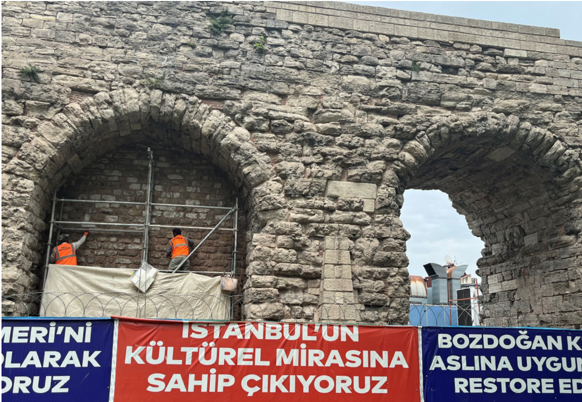
^ Fig. 4 Restoration work on the Valens Aqueduct (Source: Mariëtte Verhoeven, 2022, CC BY-NC-ND 4.0).
