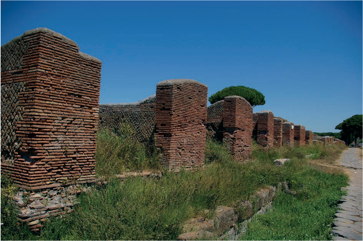
Fig 7. Building III, IV, 1-3.
