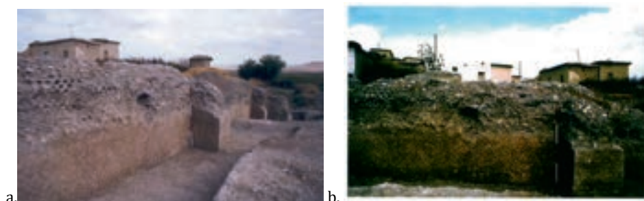
Fig. 7.36a-b. Pictures of the wall in opus caementicium with a facing in opus reticulatum, in the south-eastern side of the Lower Town, near the Urfa Gate. Source: Wagner Archive.
