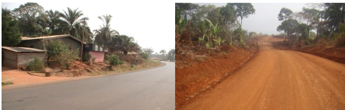
Figure 4.11: Houses and Farms affected by road construction works.
