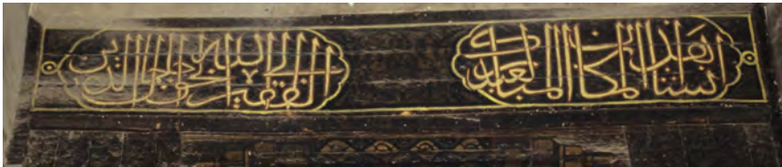
FIGURE 5.3 First part of the foundation inscription in lintel of north iwān of the Bayt al-Dhahabī first-floor qā'a in thuluth script
