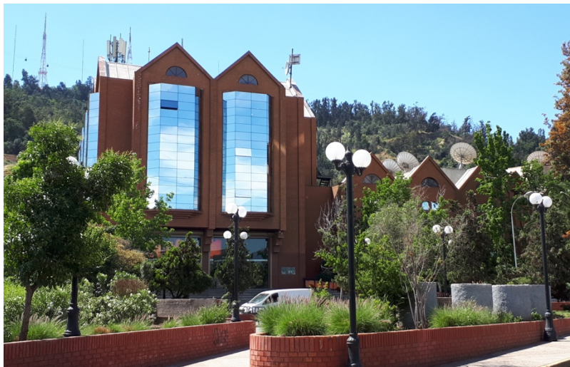
Figure 3. Canal 13's current building on Inés Matte Urrejola 848 in Santiago. San Cristóbal hill and the antennas can be seen in the background. Photo: Tomás Dodds during fieldwork.
