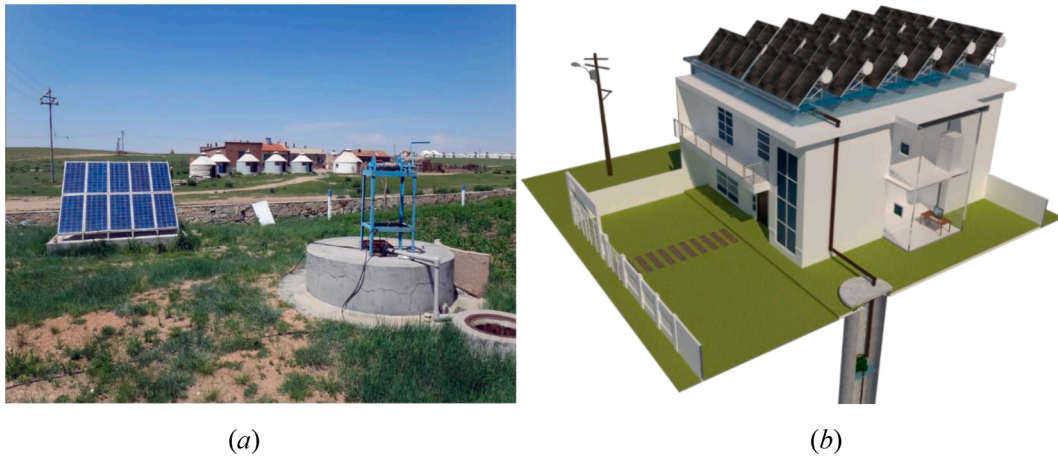
Fig. 3. (a) a PV-pump used in agricultural irrigation. [18] (b) A rendering of a household PV-PH system.
