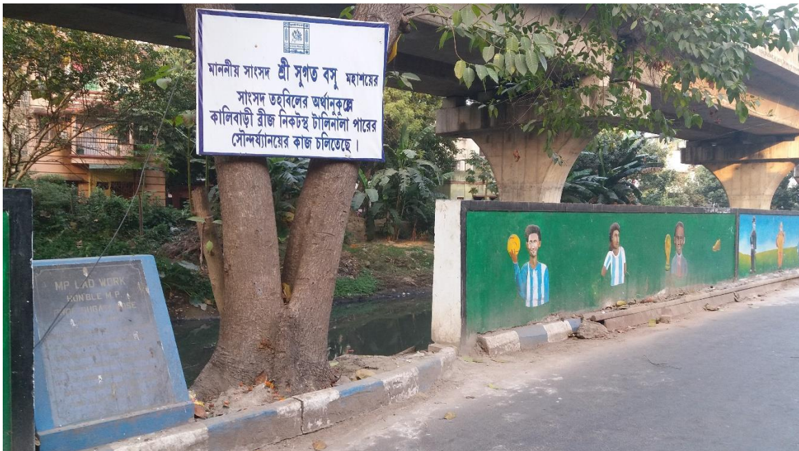
Figure 3.15. Walls have been built by the south-eastern stretch of the Pali Nala after evictions.
