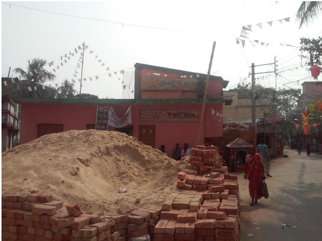
Figure 2.7. A new construction is taking place in camp I.
