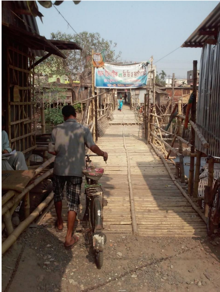
Figure 2.2. A footbridge over the Bahirdoba canal.
