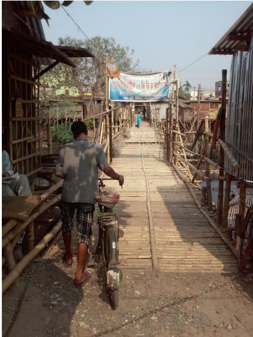
Figure 2.2. A footbridge over the Bahirdoba canal.
