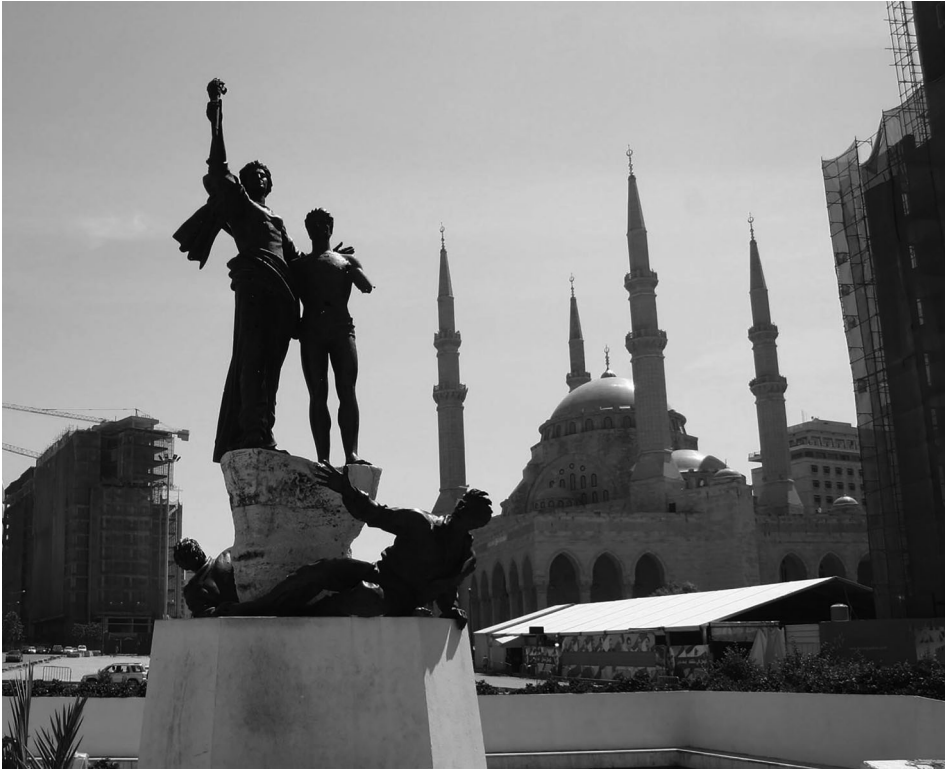
Figure 1. The tent structure of Hariri's shrine between the Martyr's Statue in the front and the Al-Amin Mosque in the back, flanked by construction sites (2014).
