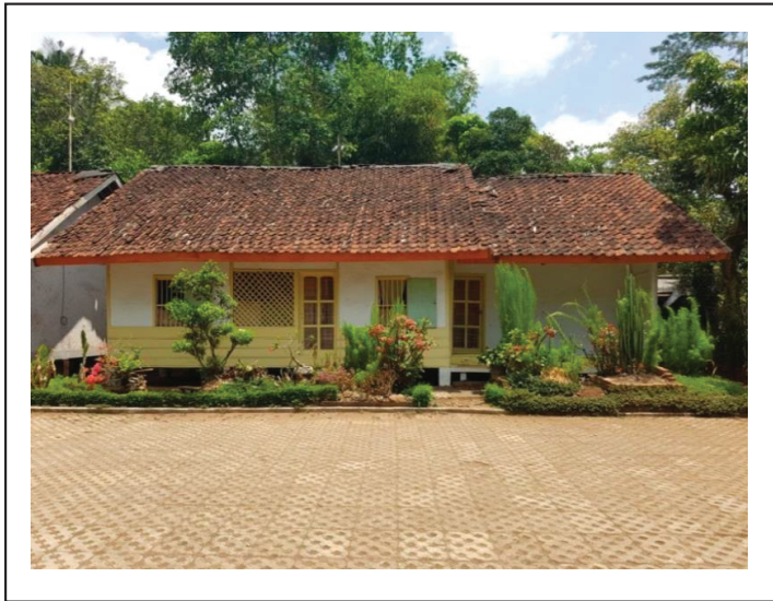
Illustration 4.2. Traditional Sundanese House in Kampung Adat Pulo (Traditional Village) Source: Photograph by M. Febriyanti (2017)
