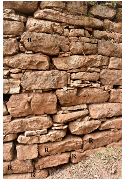
Figure 1.4b: the red limestone employed in the lower courses of the left stonion side (Photograph: A. Brysbaert).
