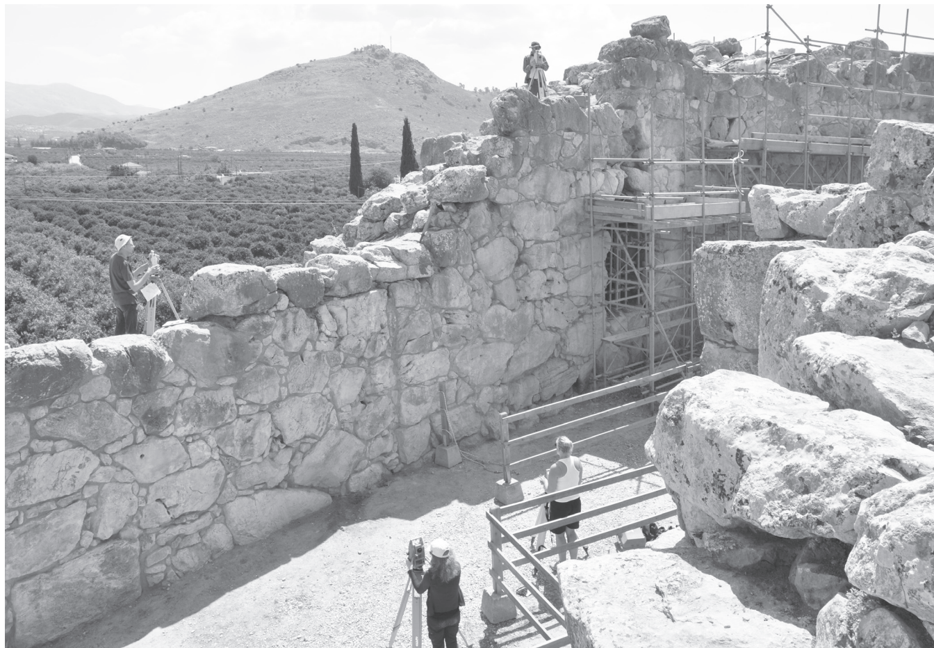
Figure 2.4. Fieldwork participants in the 3D recording of Tiryns fortification walls. Each team member needs a certain amount of space to be able to record the wall and, simultaneously, not to overlap with the work of the others. Photo: Ann Brysbaert.
