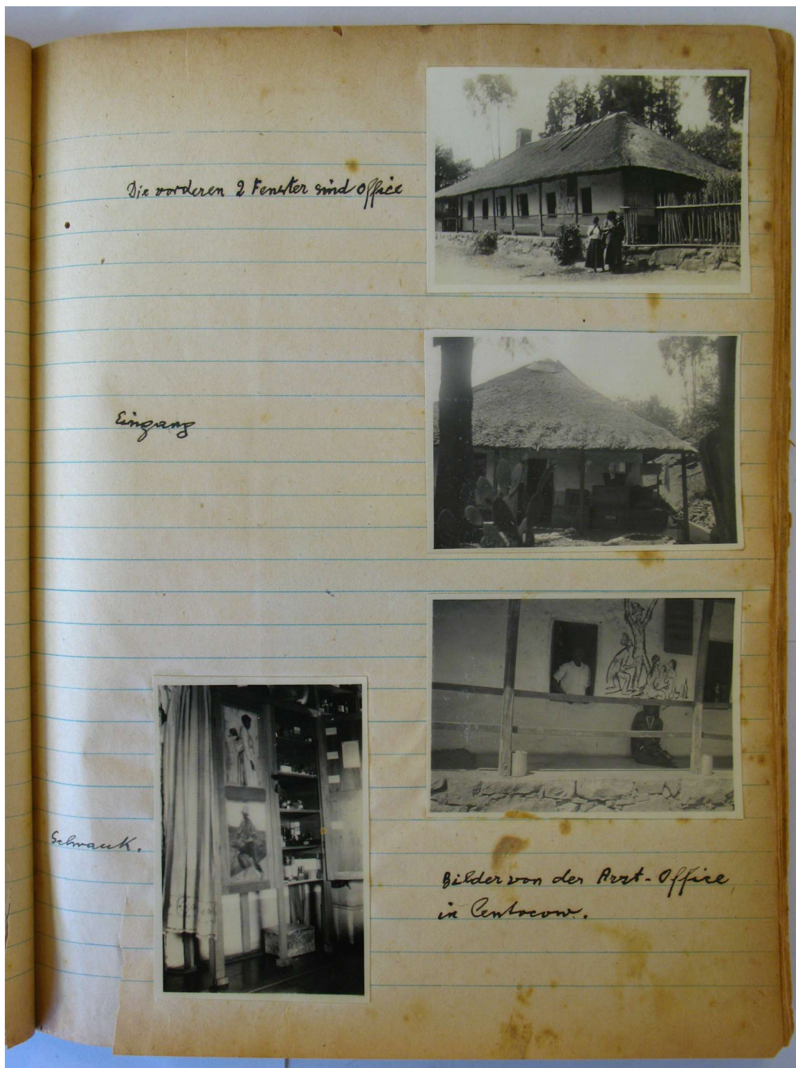
Figure 127: various photographs showing Kohler's office at Centocow. Page from one of Kohler's scrapbooks, titled "Glückliche Reise". Original captions: "[1] Die vorderen 2 Fenster sind Office; [2] Eingang; [3] Schrank; [4] Bilder von der Arzt-Office in Centocow"—"[1] The closest 2 windows belong to the office; [2] Entrance; [3] Cupboard; [4] Pictures of the doctor's office at Centocow" (KCAL).
