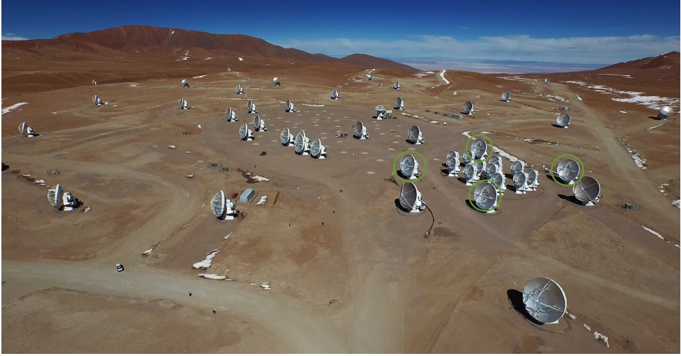
Figure 1.11: Antennas of the Atacama Large Millimeter/submillimeter Array (ALMA). Fifty of these antennas have 12 m diameters and make up the “12 m array”, used for sensitive, high-resolution imaging. Green circles in this image mark four additional 12 m antennas that are used for total power observation (the “TP array”), and interior to those are twelve closely spaced 7 m antennas (the “7 m array”). The 7 m and TP arrays enhance wide-field imaging of extended structures and are collectively referred to as the Atacama Compact Array.
