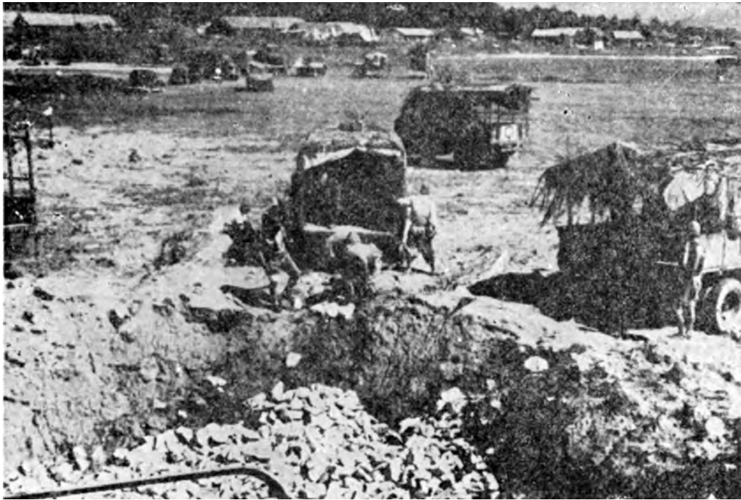
The Repair of Bomb Craters
