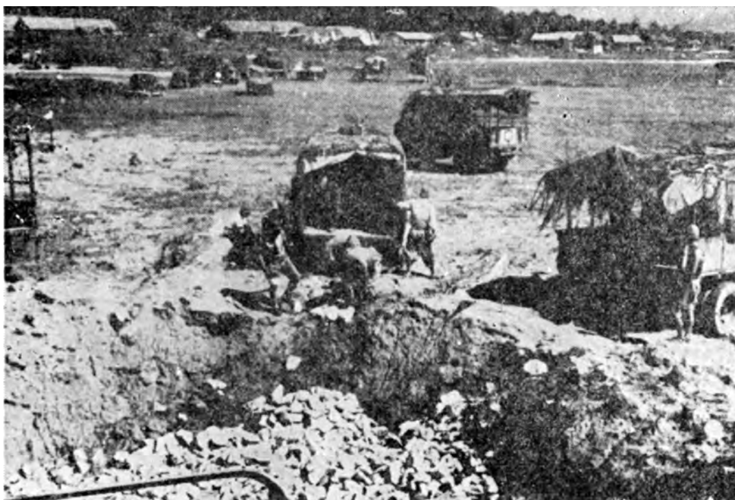
The Repair of Bomb Craters
