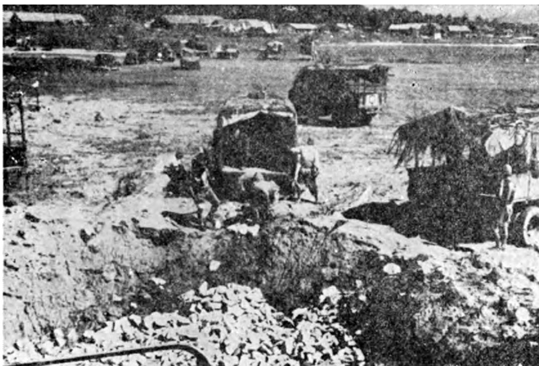
The Repair of Bomb Craters
