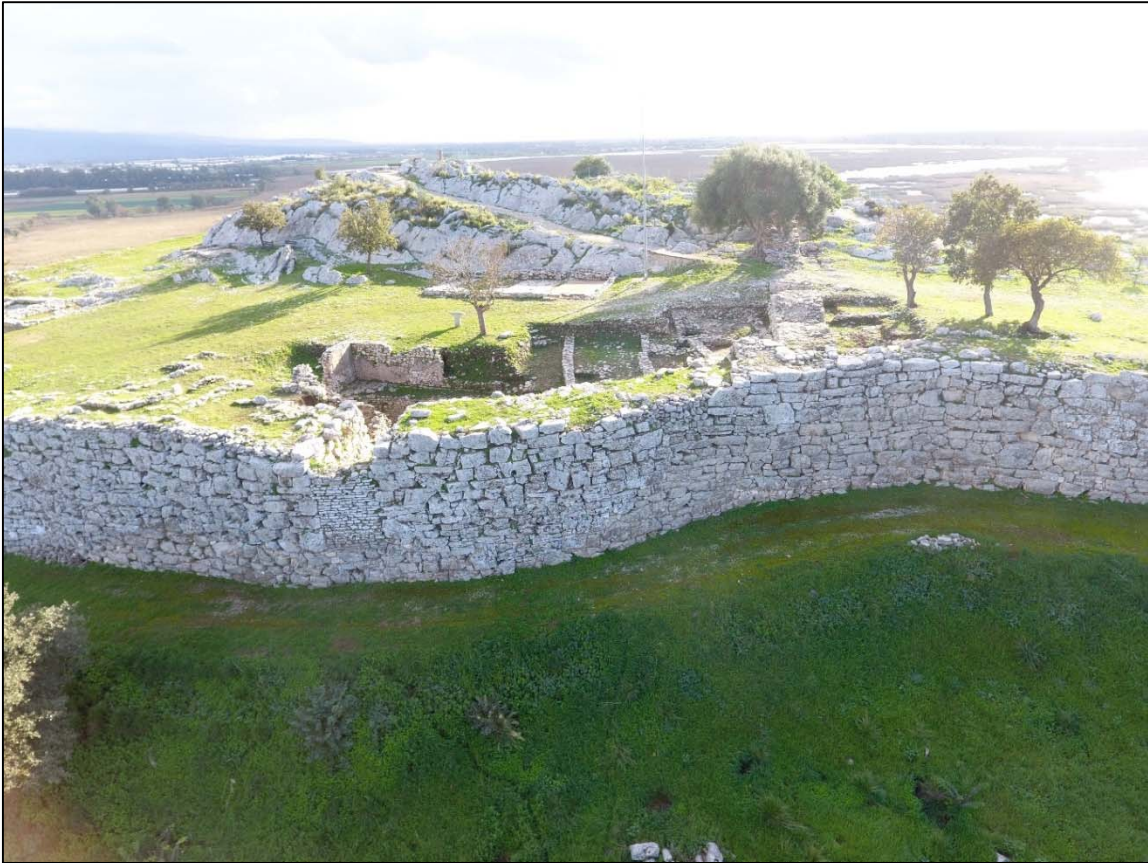
Figure 4.7 Section of the fortification wall at Teichos Dymaion. Just left of the middle, the section with smaller stones can be seen, this is the walled up Middle Gate. Furthermore, the image shows how much of the interior face of the fortification wall is still buried (photograph taken by Ann Brysbaert and Jari Pakkanen).
