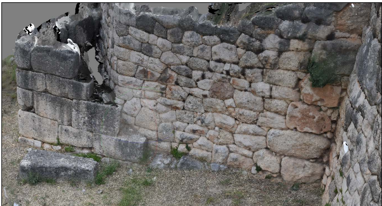
Figure 3.6 View on the backside of the bastion at the Lion Gate, Mycenae (textured 3D model by author). The cut blocks on the left form a separate façade around the wall (note that this section of wall might not be cyclopean). It also shows the somewhat irregular shape and size of these conglomerate blocks, as mentioned by Küpper, which makes that he does not consider them as true ashlar.
