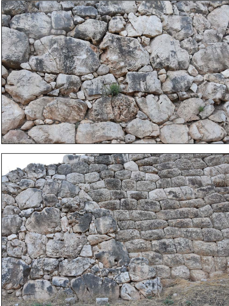
Figure 3.2 Top: Cyclopean-style wall. Part of the fortification at Mycenae. Bottom: difference between the cyclopean-style section (left) and the later Hellenistic polygonal-style section (right). Note the well-fitting blocks in the Hellenistic section. Each block had to be cut specifically to fit. Also note that many blocks on the left are quite a bit larger than those on the right (photographs by author).
