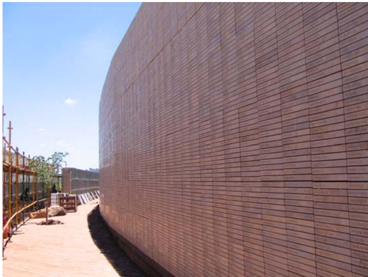
Photo 7.4 Wall of Names Freedom Park, Salvokop (Tshwane), photographed in December 2008.
