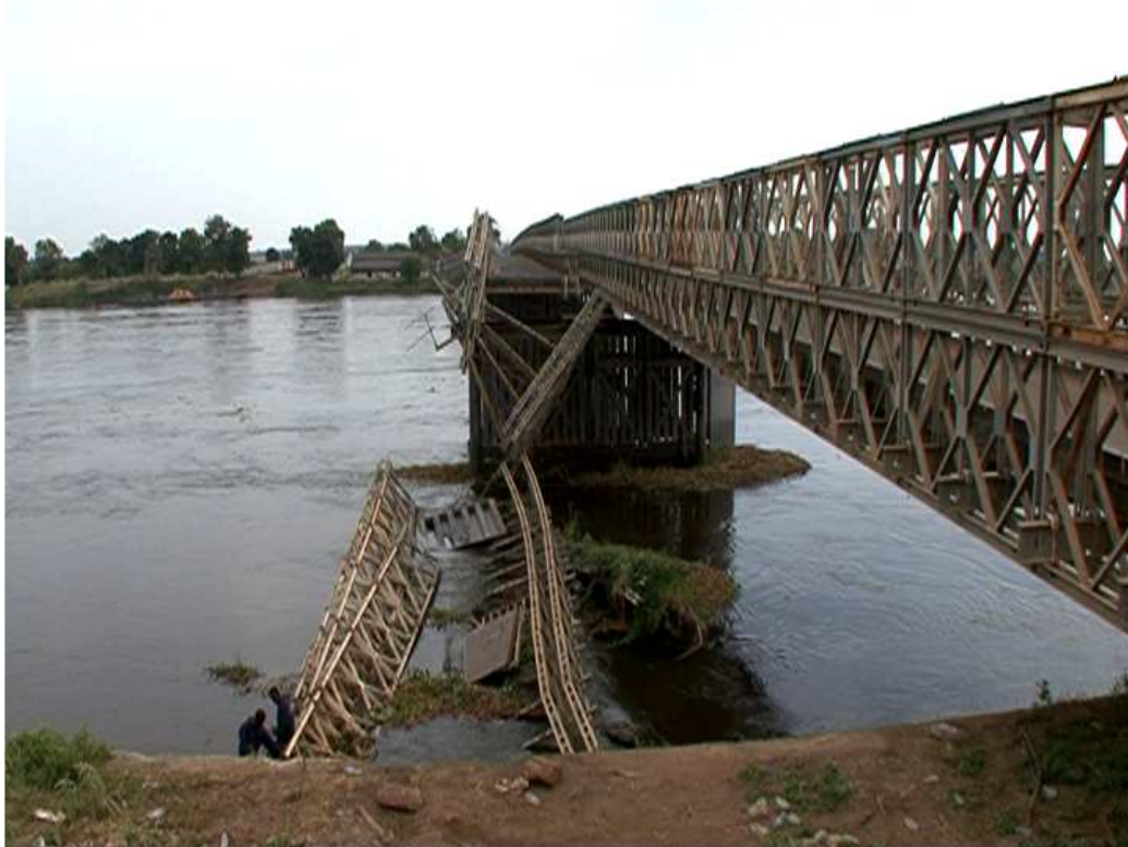
Picture 30: Bridge over the Nile, Juba
